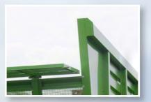
Hood-type end profile New top flange designed as a hood-type profile to prevent trickle loss.
